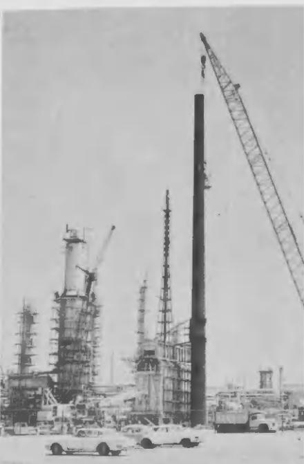
At left, the old section of the 83-ft high splitter tower before removal. At right, preparations are made to take down the furnace stack.
